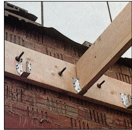
Figure 4. Floor joists are hung from ledgers that are bolted to an integral bond beam in the brick wall.
