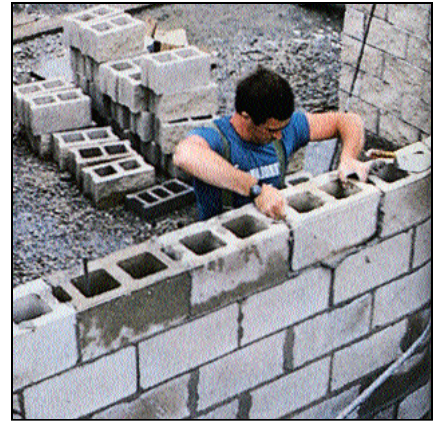
Figure 7. The architectural face of the split rib concrete block is turned inward to give the basement walls an appealing interior finish that needs no painting or other treatment.
