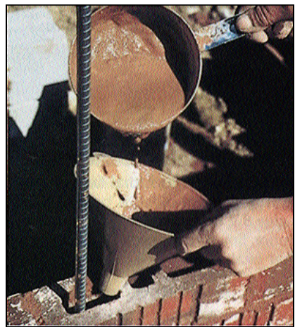
Figure 3. Using small buckets, workers then pour grout into the cores a few courses at a time. Pumping grout in high lifts could reduce cost more.
